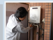
給湯器故障取替
